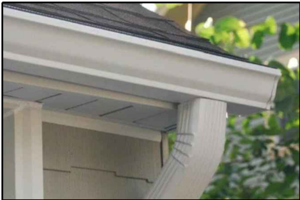
GUTTERS AND DOWNSPOUTS: PREFINISHED WHITE 5" K STYLE/ 2X3 DOWNSPOUTS
